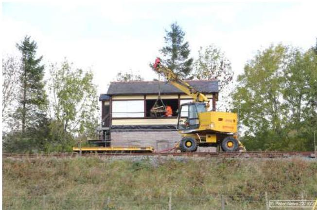
*Windows being lifted into place on the signal box Photo : PN*
