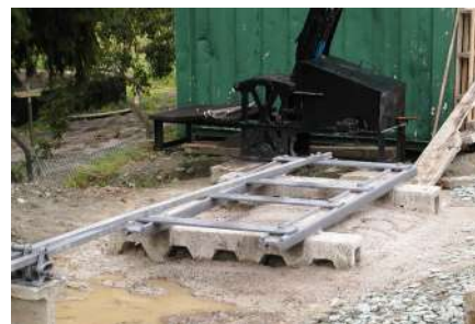
Groundframe base awaiting the frame seen in the background Photo: PR
