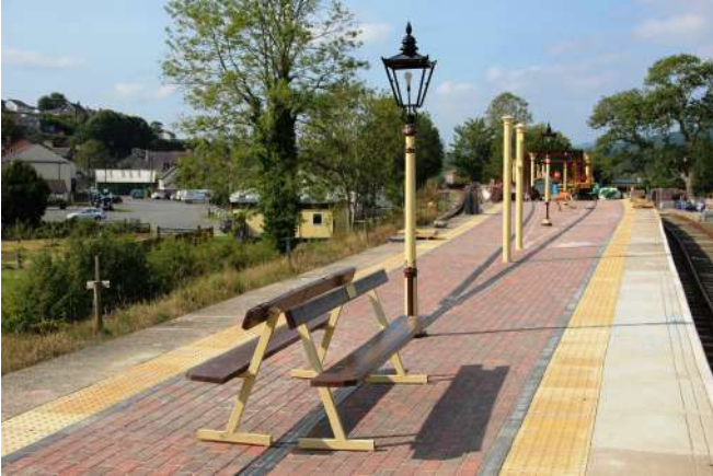
Completed platform surface showing gentle slope to the centre and drains Photo : PR
