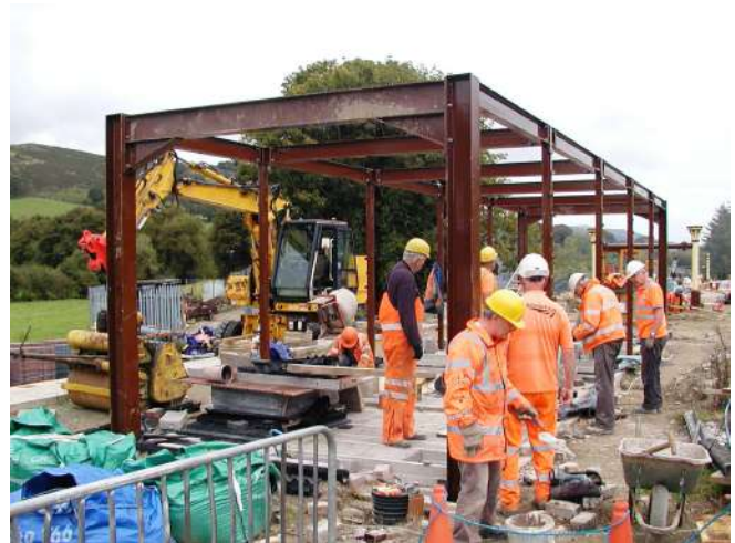
Bricking and concrete gang filling in round the posts
