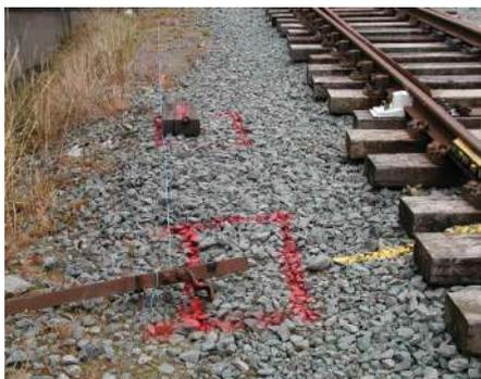
*Position for point crank block Photo: PR*
