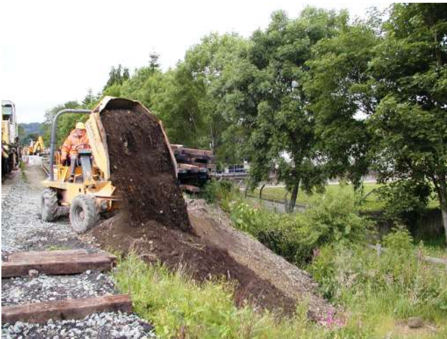
Tipping soil to widen the embankment Photo : PR
