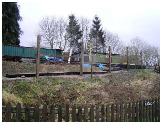
Post and railed walkway up the ramp Photo : PR
