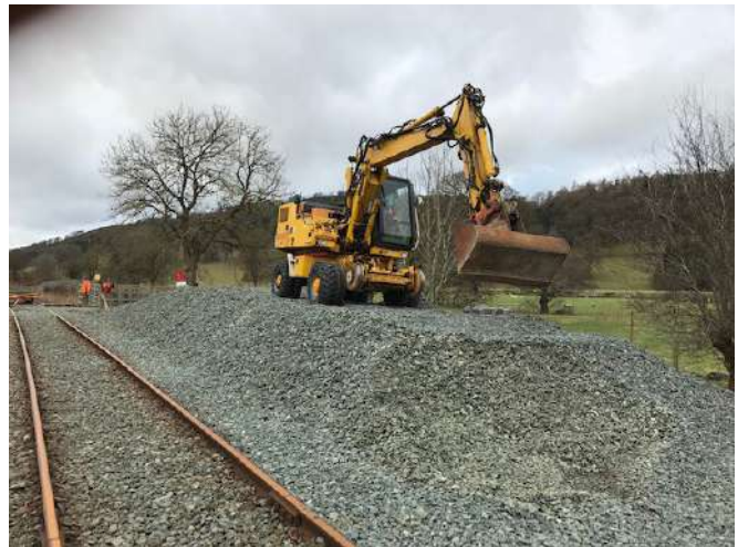
RRV on the Ballast stack
