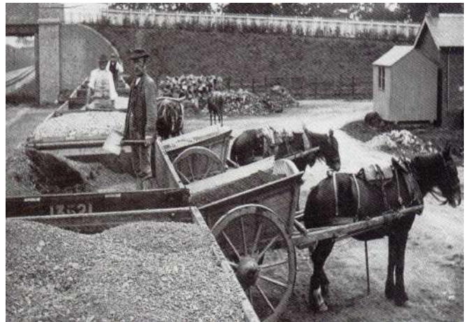
Trans-shipping track ballast at Charwelton depot Photo: SWA Newton Leicester County Record Office Archive
