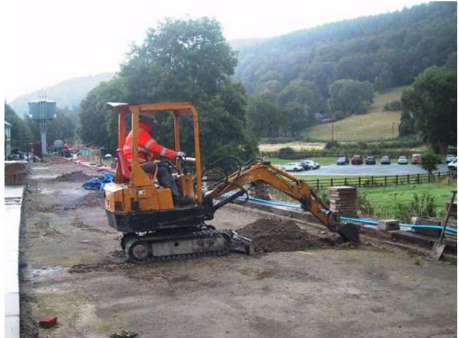
*Joel Scott on the Nissan mini digger preparing a trench for large drain pipes* Photo : PR
