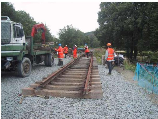
*New track panel added to the main line to facilitate the arrival of ballast from the Bonwm stockpile
